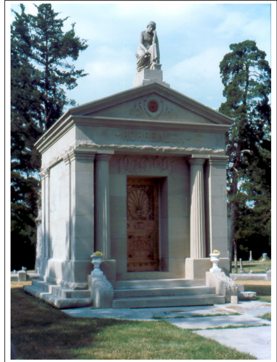
In 1901, Rohrbaugh built a beautiful mausoleum in Hope Cemetery where he, his wife and son are interred. George Washburn was the architect.
