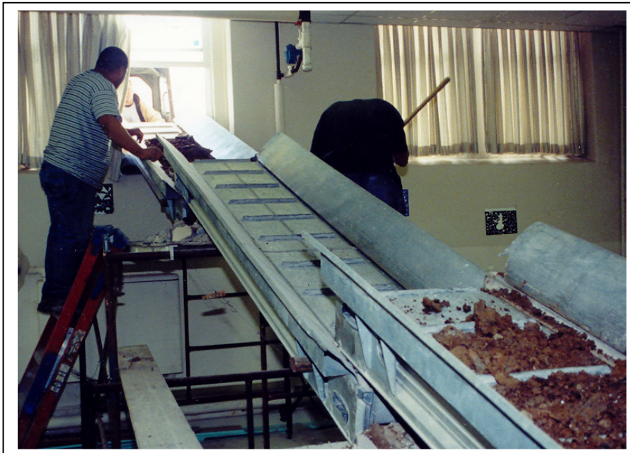
Two photos showing the remodeling work. The left photo shows the conveyors moving the dirt removed for the elevator pit out of the building.
