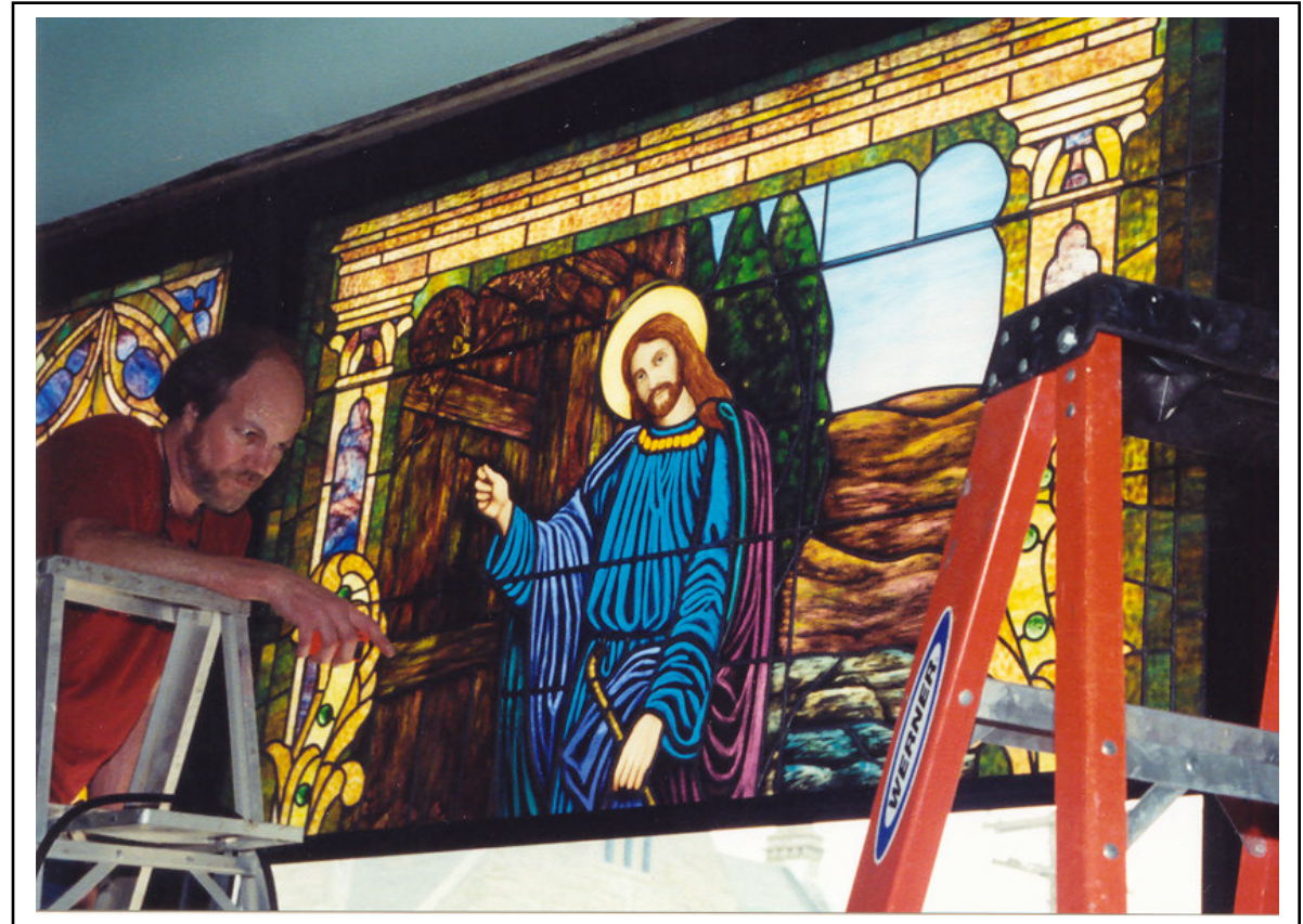
Cliff Mayfield of Karen Hendrix & Associates installing the replacement "Jesus Knocking" stained glass window.
