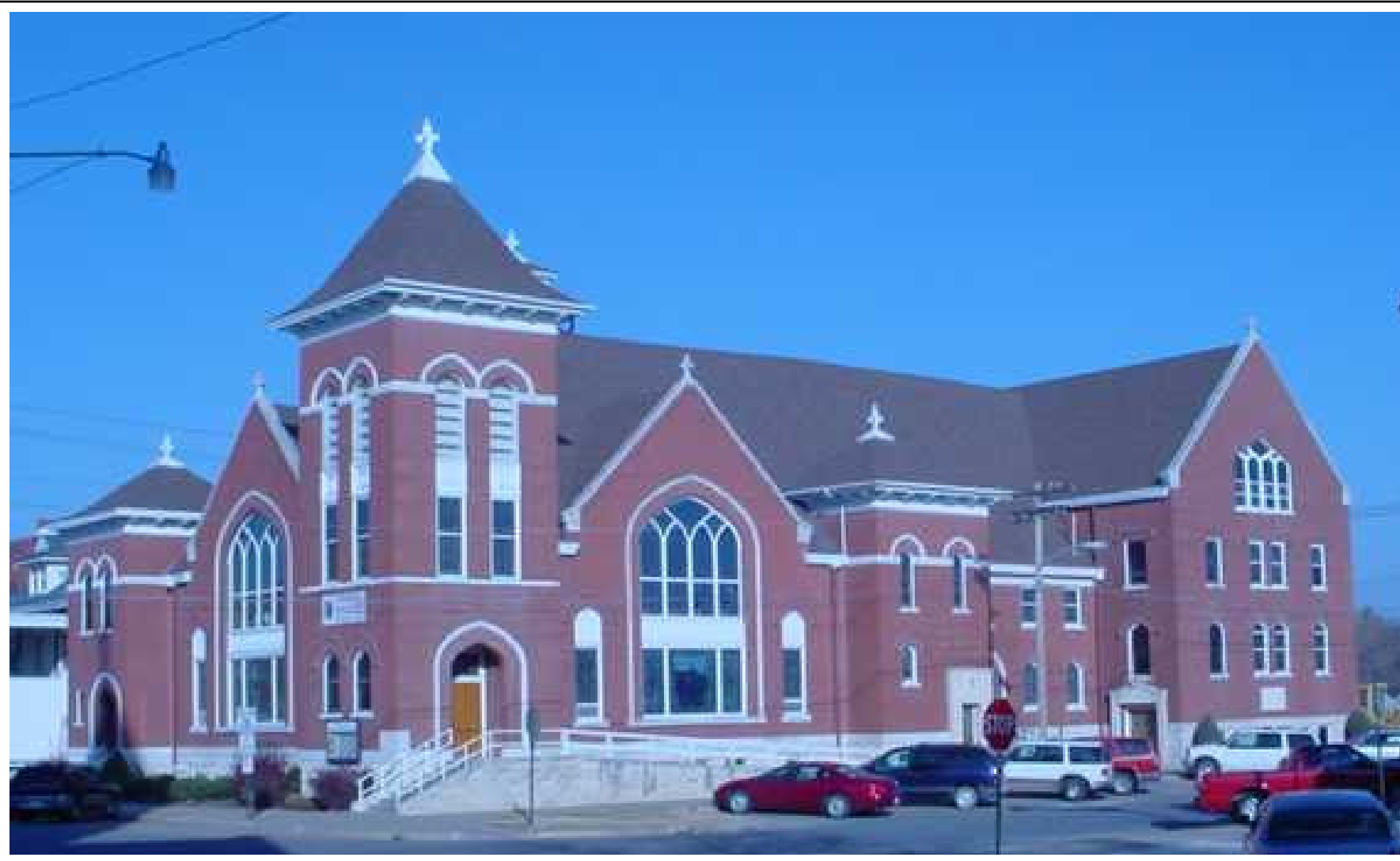
The Church today showing the ramp added in 1981.
